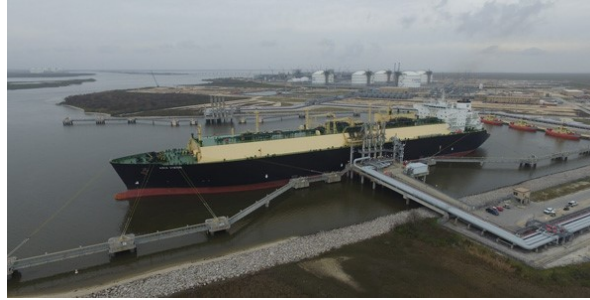
Loading of the first commissioning cargo at Sabine Pass LNG Terminal in February 2016 | Cheniere Energy
